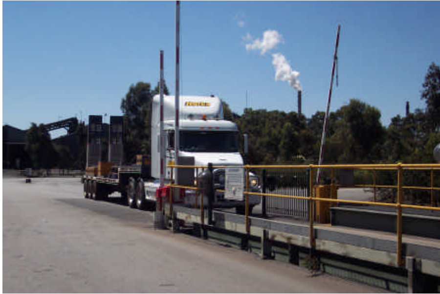
Figure 16: Sample of a full length weigh bridge capable of split weighing axles accurately due to the long flat approach.
